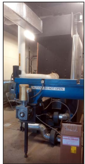
(Left) Front of the boiler where ash is deposited and (Right) back of the boiler where wood chips are fed via auger from the storage room.
