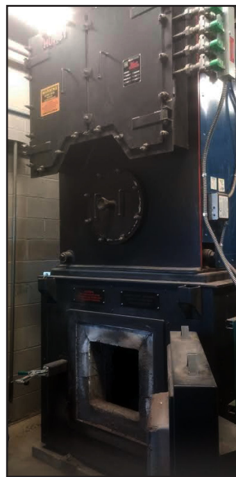
(Left) Front of the boiler where ash is deposited and (Right) back of the boiler where wood chips are fed via auger from the storage room.
