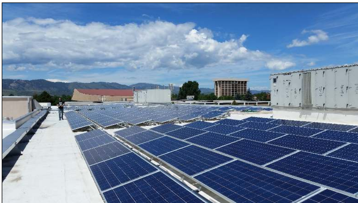
A 545 kW solar array located on the Student Recreation Center at CSU
