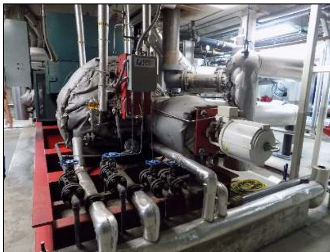
This 800 kW Steam Turbine Generator at the Main Campus Central Heating Plant recovers enough waste heat energy to meet 5% of the campus peak electrical load
