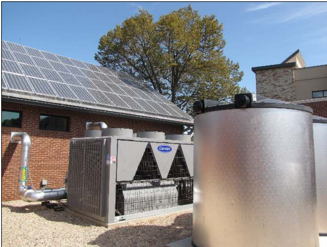
Thermal storage tanks & solar photovoltaic panels at the Academic Village Residence Hall
