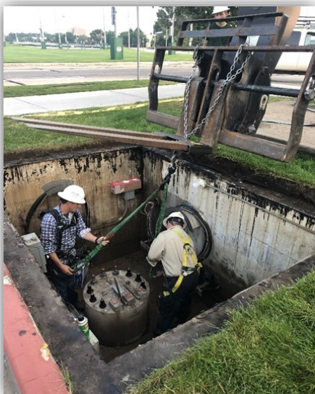
Old switch ready to be removed
